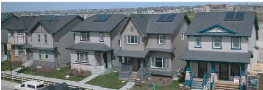
Drake Landing Solar Community homes collect solar energy with two EnerWorks solar collectors for domestic hot water.
