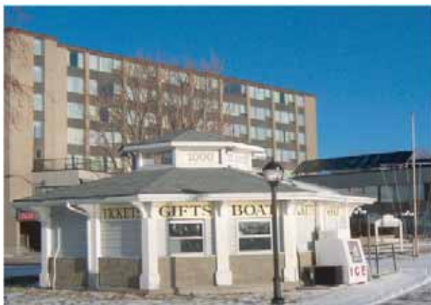
Confederation Place Hotel on the historic waterfront in Kingston, Ontario. Solar collectors can be seen at right, on top of hotel conference center.
