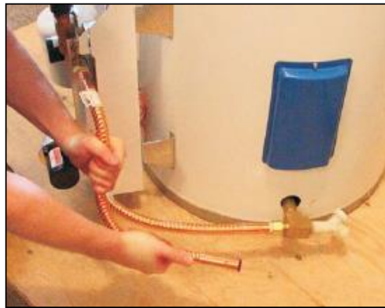
Fig. 4.5.1 – Fabrication of heat trap using a flexible corrugated pipe to cold mains inlet. Using two hands bend pipe down and back (not included).
