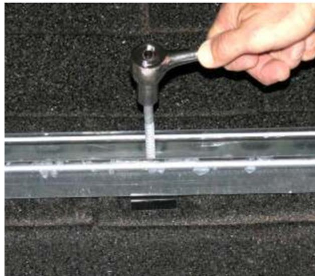
Fig. 5.2.5 – Securing C-channel with lag-bolts.
