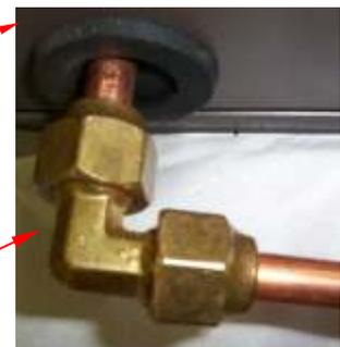
Fig. 6.5.2 – Flare fitting 90° elbow connects line-set to collectors (to be insulated after pressurizing heat-transfer fluid).
