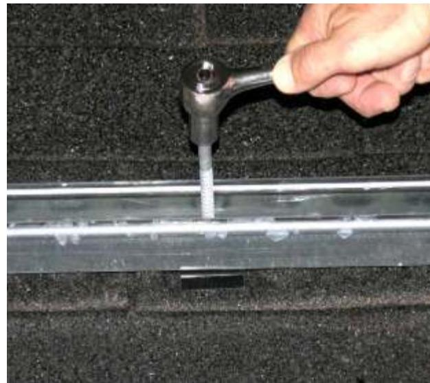
Fig. 5.2.5 – Securing C-channel with lag-bolts.
