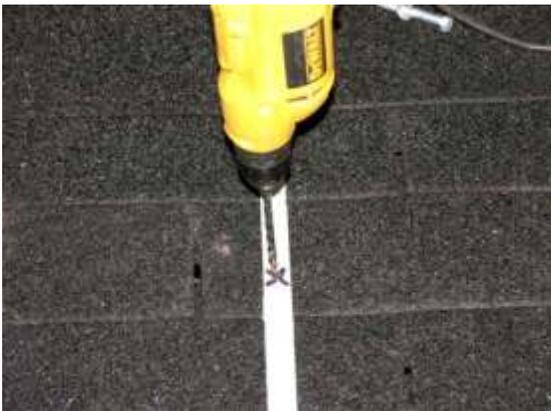
Fig. 5.2.3 – Pre-drill lag-bolt hole.
