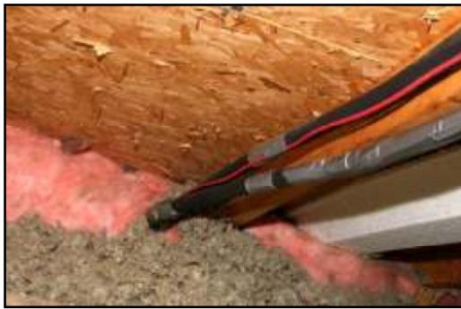
Fig. 4.2.2 – Line-set and control-wire in attic.
