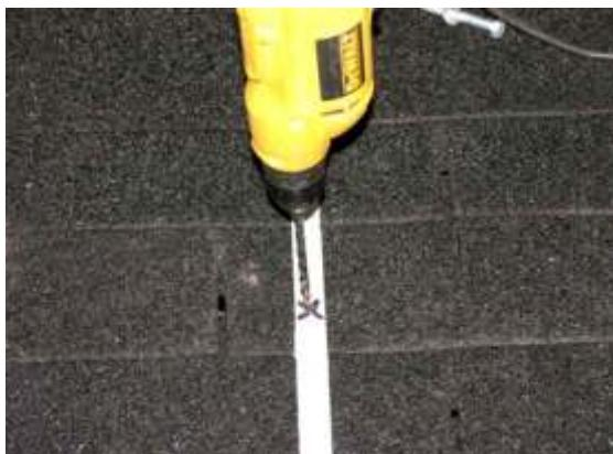
Fig. 5.2.3 – Pre-drill lag-bolt hole.
