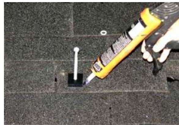
Fig. 5.2.4 – Roof-sealant application.
