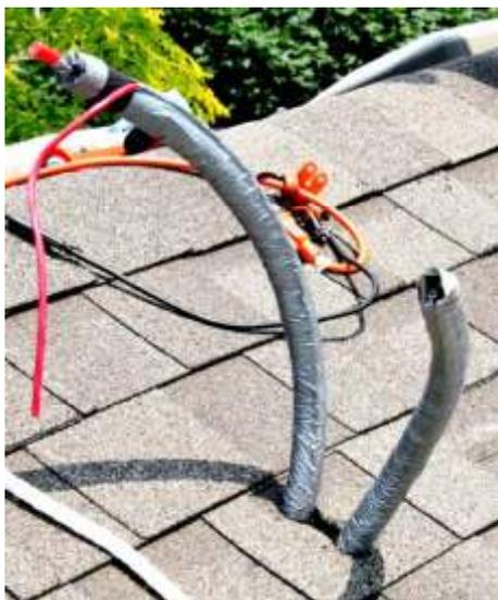
Fig. 5.4.1 – Line-set and control wire protected with tape.
