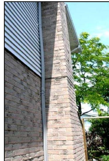
Fig. 4.2.3 – Exterior line-set in downspout
