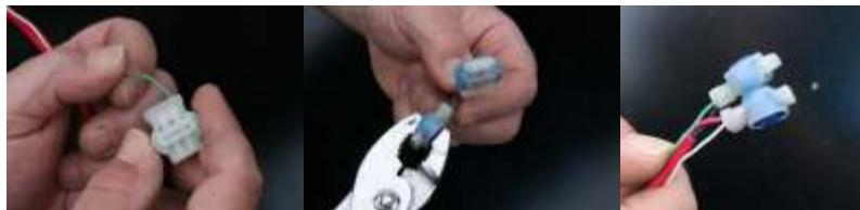
Fig. 6.5.1 – To make thermistor/control-wire connections, insert unstripped conductors into IDC and squeeze with pliers.
