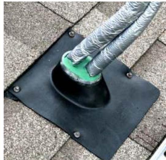
Fig. 5.4.3 – Finished line-set boot flashing.
