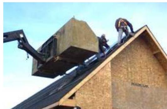
Fig. 6.2.3 – Lifting and securing collectors using forklift boom.
