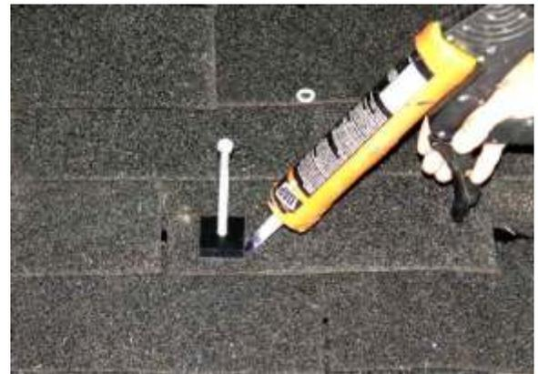
Fig. 5.2.4 – Roof-sealant application.
