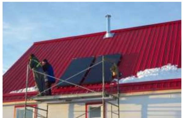
Fig. 6.2.4 – Scaffolding used for lifting and as work platform.
