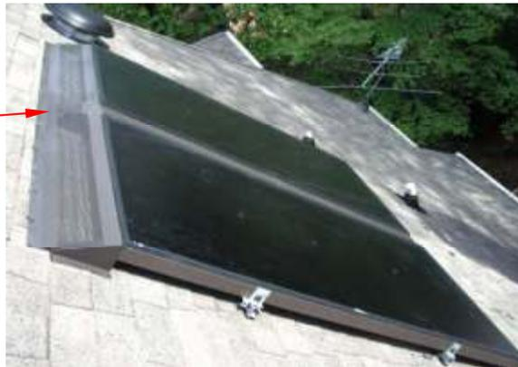
Fig. 7.3.1 – Two collectors with center-flashing and leaf-guard.
