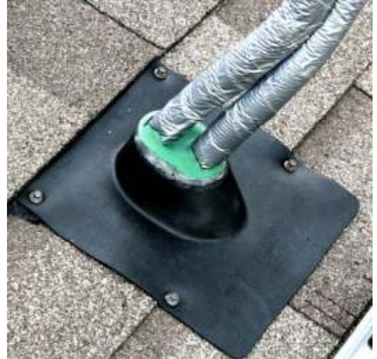
Fig. 5.4.3 – Finished line-set boot flashing.
