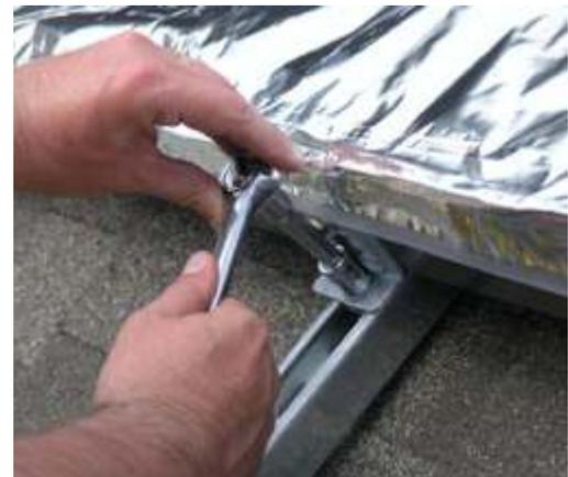
Fig. 6.3.1 – Securing collector with ratchet and extension.
