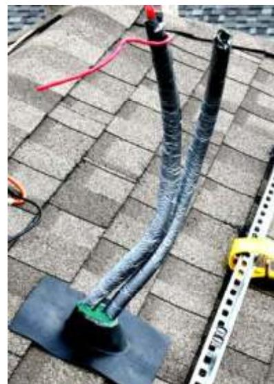
Fig. 5.4.2 – Boot flashing before insertion under shingle.
