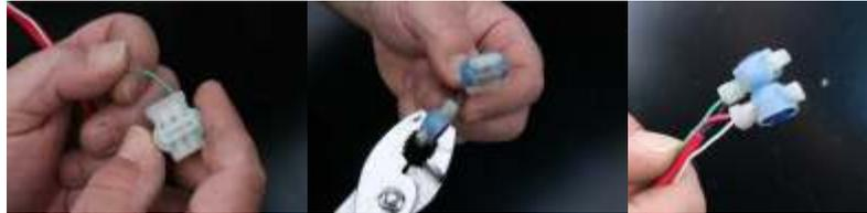
Fig. 6.5.1 – To make thermistor/control-wire connections, insert stripped conductors into IDC and squeeze with pliers.
