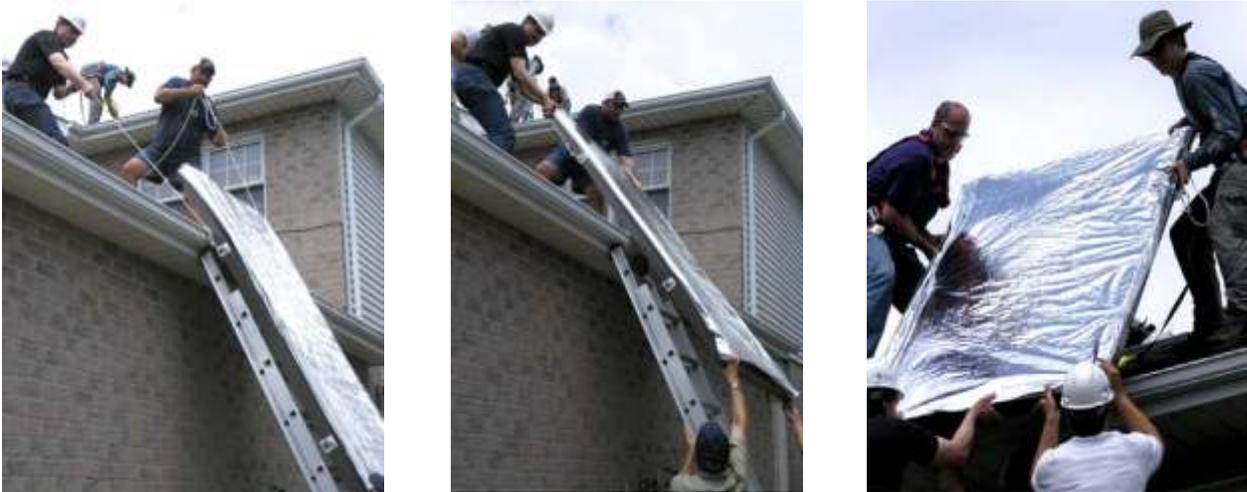
Fig. 6.2.6 – Lifting collector to roof using ladder and lines.
