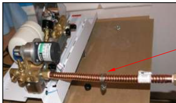
Fig. 4.2.1 – Flexible pipe connected to Energy Station. Hose clamp ready to attach thermistor.
