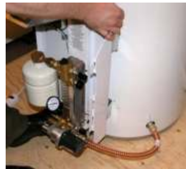
Fig. 4.2.7 – Securing Energy Station.
