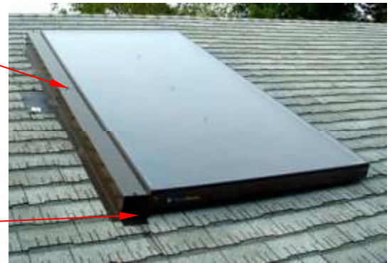
Fig. 6.1.1 – Collector side-flashing. Note roof-penetration boot under side-flashing.
