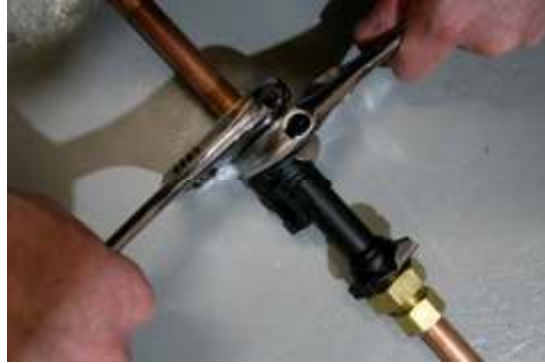
Fig. 4.5.7 – Use two wrenches to tighten compression nuts.
