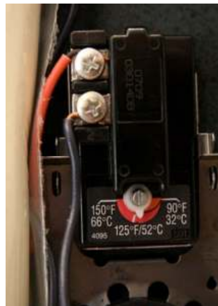
Fig. 4.10.5 – Connect red and black wires to lower thermostat terminals. Set thermostat to 120 °F (50 °C).
