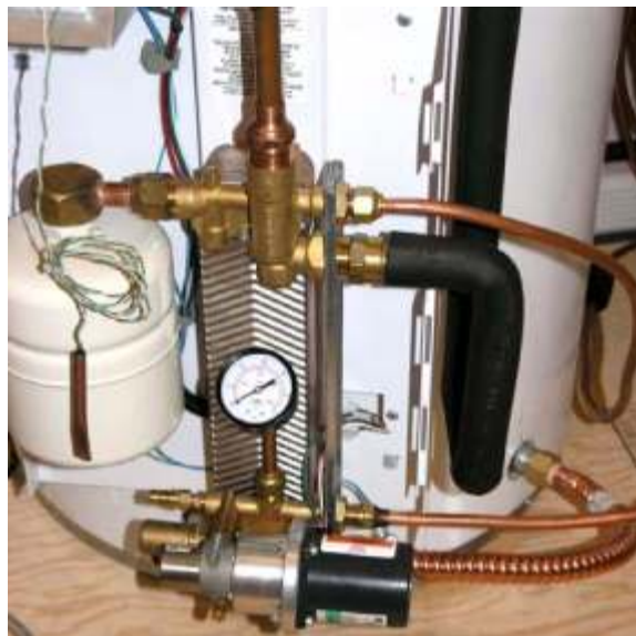
Fig. 4.9.1 – Line-set connections to Energy Station. Note: For clarity, line-set is not insulated. Proper installation must have insulated line-set to prevent heat loss and to limit burn risk.
