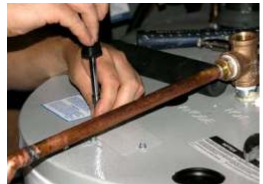
Fig. 4.10.1 – Remove connection cover plate.
