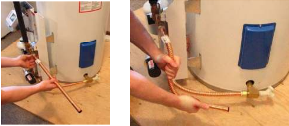
Fig. 4.5.8 – Thread and tighten 24" (60.96 cm) flexible corrugated pipe to cold mains inlet. Using two hands, bend pipe down and back.
