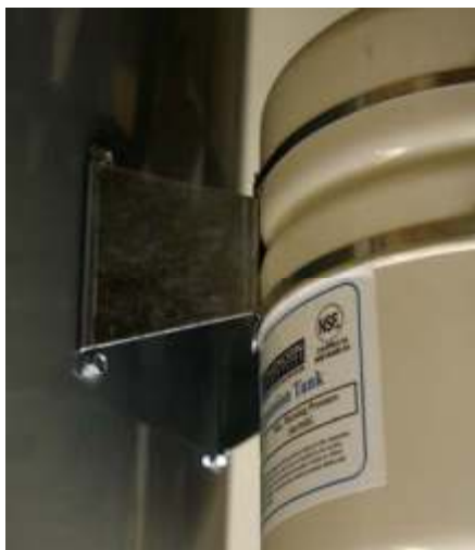
Fig. 4.9.2 – Supplemental expansion tank mounted to tank with self-drilling screws.
