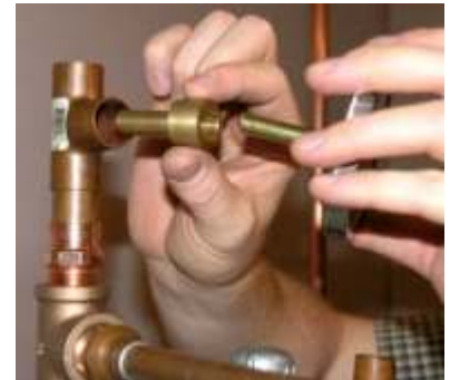
Fig. 4.3.3 – Remove thermometer from well
