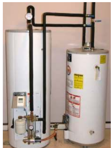
Fig. 4.8.1 – All pipes and fittings insulated to limit heat loss and prevent condensation.
