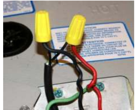
Fig. 4.10.3 – Connect over-temperature wire to tank wires.
