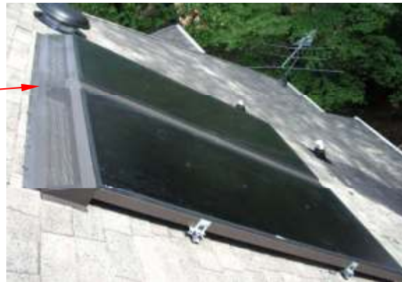
Fig. 6.3.1 – Two collectors with center-flashing and leaf-guard.
