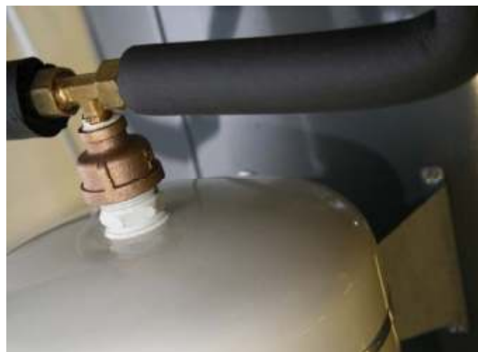
Fig. 4.9.3 – Supplemental expansion tank in line from collector to top of heat exchanger.
