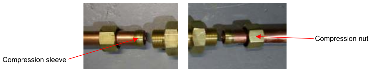
Fig. 4.5.6 – Slide compression nuts and sleeves over 1/2" pipe. Insert pipes into fittings.
