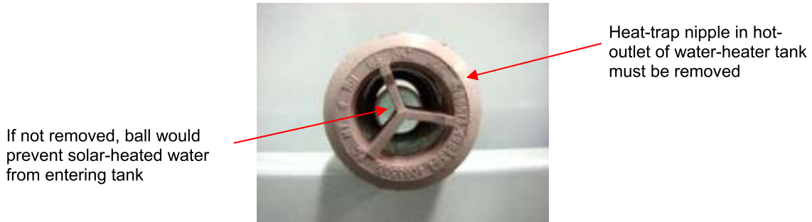
Fig.2.4.1 – Heat-trap nipple or gasket must be removed from solar storage tank.
