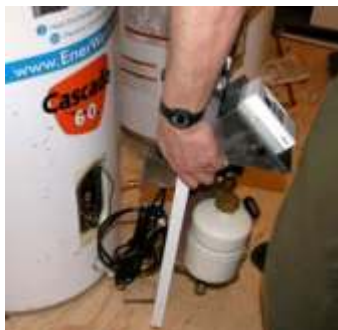
Fig. 4.2.6 – Positioning Energy Station.
