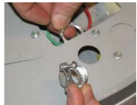
Fig. 4.10.2 – Punch out insert and install cable-clamp.
