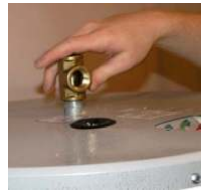
Fig. 4.3.1 – Brass tee connected to top of solar storage tank
