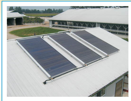
300 cow dairy farm: This solar thermal system near Innerkip supplies about 1200 liters of hot water per day to wash the milk tanks and 6 milking robots.
