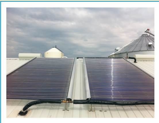
Broiler and hog farm: The solar hot water system is used for radiant floor heat, domestic hot water and to heat a fat tank used for process feed.
