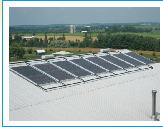
2000 liters of hot water: 16-collector system near Bright provides hot water demand for 200 plus cow dairy farm milking 3 times per day. Excess hot water is fed back to the cows.
