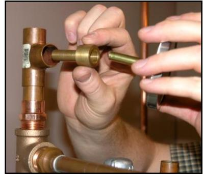
Fig.4.3.3 – Remove thermometer from well
