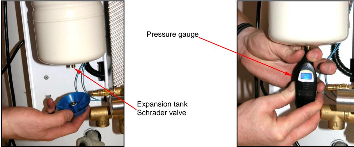
*Fig.4.2.3 – Expansion tank Schrader valve and pressure measurement*
