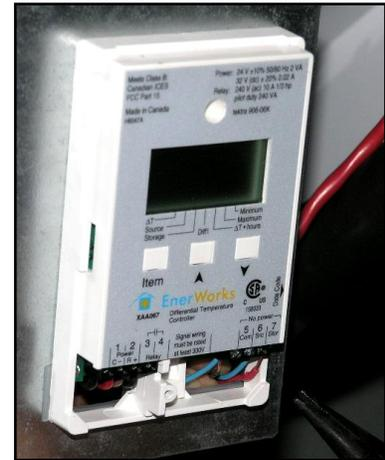
*Fig. 4.11.1 – Controller with cover removed*
