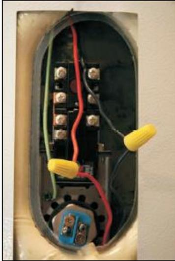
Fig. 4.10.1.4 – Connect wires to bypass upper thermostat.
