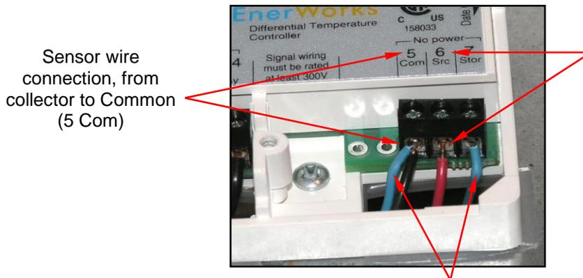
Sensor wire connection, from collector to Common (5 Com)
