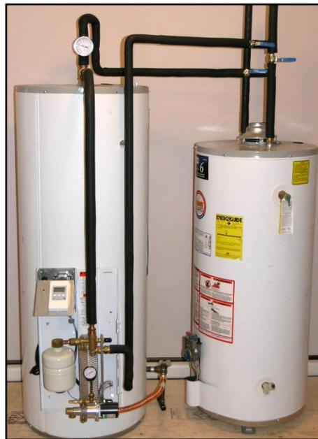
*Fig.4.6.1 – All pipes and fittings insulated to limit heat loss and prevent condensation.*
