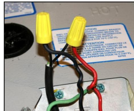
*Fig.4.10.1.3 – Connect over-temperature wire to tank wires.*
