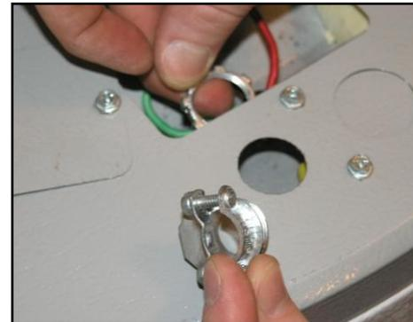
*Fig.4.10.1.2 – Punch out insert and install connector nut*
