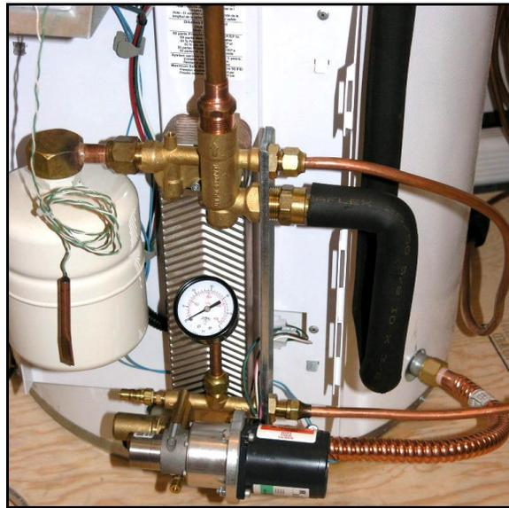
*Fig.4.9.1.1 – Line-set connections to Energy Station. Note: For clarity, line-set is not insulated. Proper installation must have insulated line-set to prevent heat loss and to limit burn risk.*
