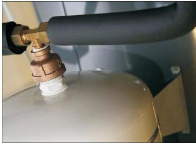
*Fig. 4.9.2.2 – Supplemental expansion tank in line from top of heat exchanger to collector.*
