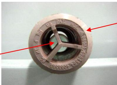
Heat trap nipple in hot-outlet of water heater tank must be removed
