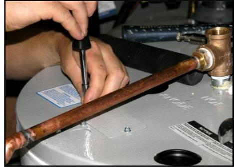
*Fig.4.10.1.1 – Remove connection cover plate*
