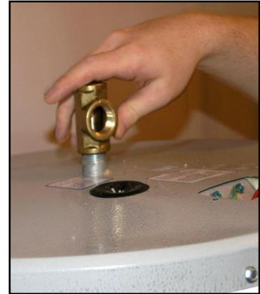
Fig.4.3.1 – Brass tee connected to top of solar storage tank
