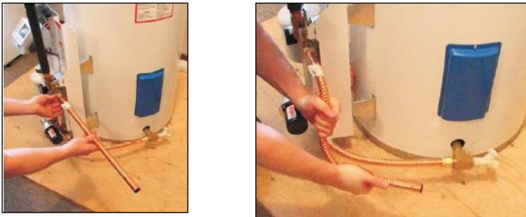
Fig. 4.5.1 – Fabrication of heat trap using a flexible corrugated pipe to cold mains inlet. Using two hands bend pipe down and back (not included).
