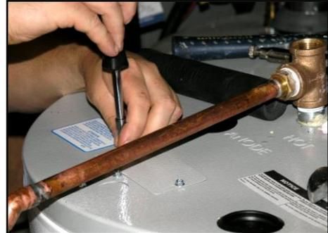
*Fig.4.10.1.1 – Remove connection cover plate*
