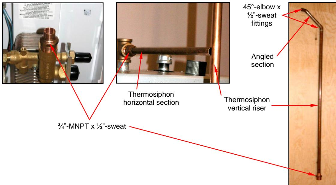
Fig.4.3.2 – Thermosiphon loop – horizontal and angled sections and vertical riser.
