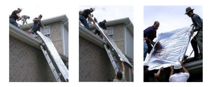
Fig. 6.2.6 – Lifting collector to roof using ladder and lines.
