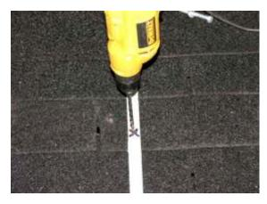
Fig. 5.2.3 – Pre-drill lag-bolt hole.
