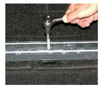
Fig. 5.2.5 – Securing C-channel with lag-bolts.
