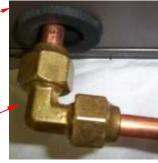
Flare fitting 90° elbow (to be insulated)
