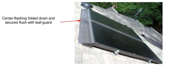
Fig. 7.3.1 – Two collectors with center-flashing and leaf-guard.
