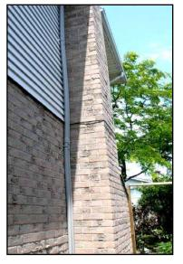
Fig. 4.2.3 – Exterior line-set in downspout
