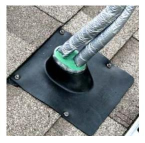
Fig. 5.4.3 – Finished line-set boot flashing.
