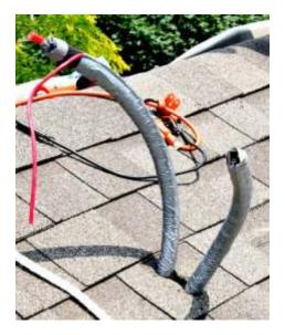
Fig. 5.4.1 – Line-set and control wire protected with tape.
