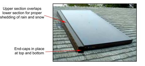
Fig. 7.1.1 – Collector side-flashing. Note roofpenetration boot under side-flashing.
